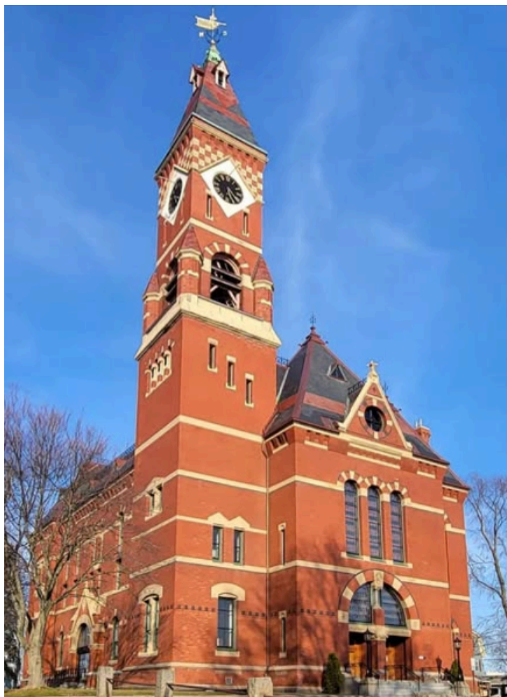
Abbot Hall in Marblehead is heated and cooled by geothermal energy.
